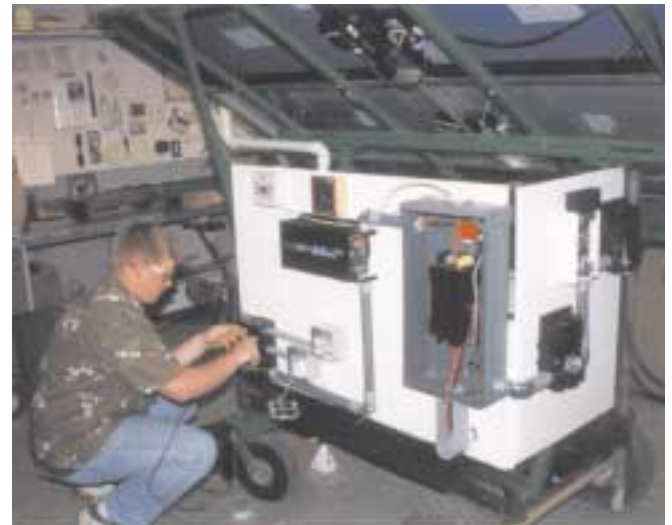
Bret wiring the AC distribution box. We installed two 15 amp circuits with four duplex outlets each.
