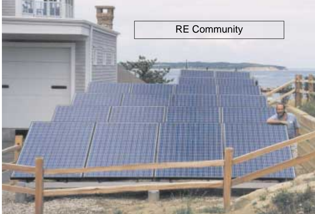
Postmaster Fred Leeder with the 6 KW array at the Block Island Post Office.
