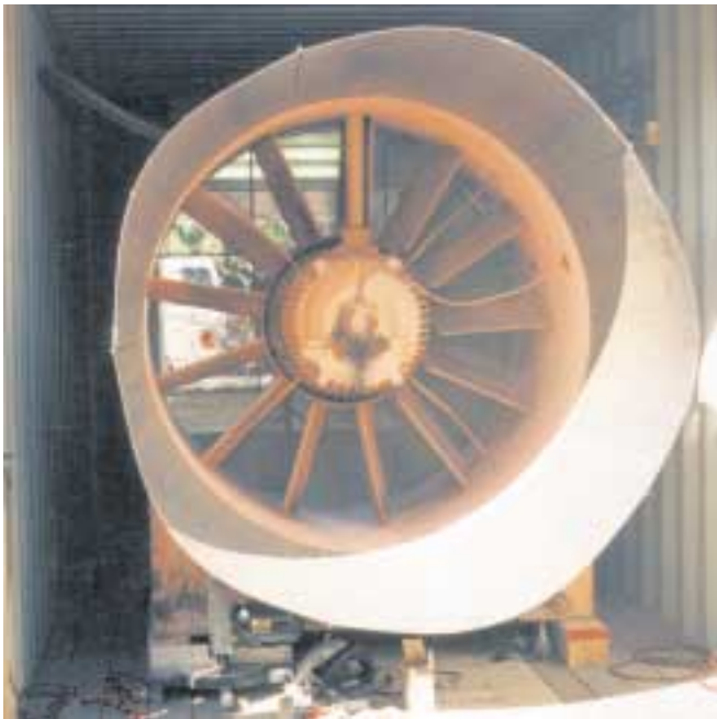
The 480 VAC, three-phase, 65 hp fan at the exhaust end of the wind tunnel uses more power than the rest of the factory.
