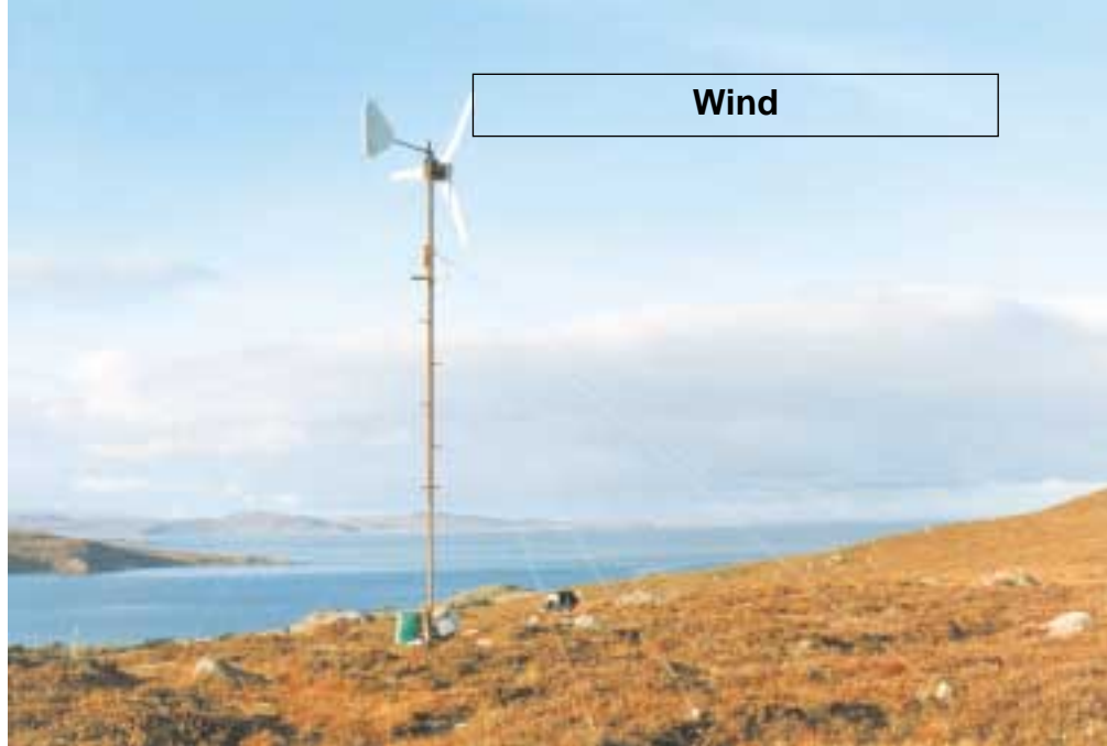
One of Hugh's home-built wind generators in Scoraig Scotland. The alternator is built from the brake drum of a truck.
