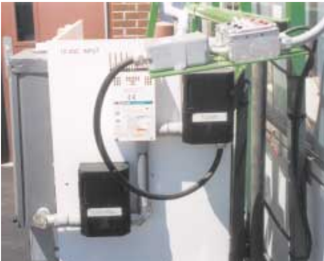
The PV junction box and two PV switch boxes. Meter probe jacks allow easy individual amperage readings.
