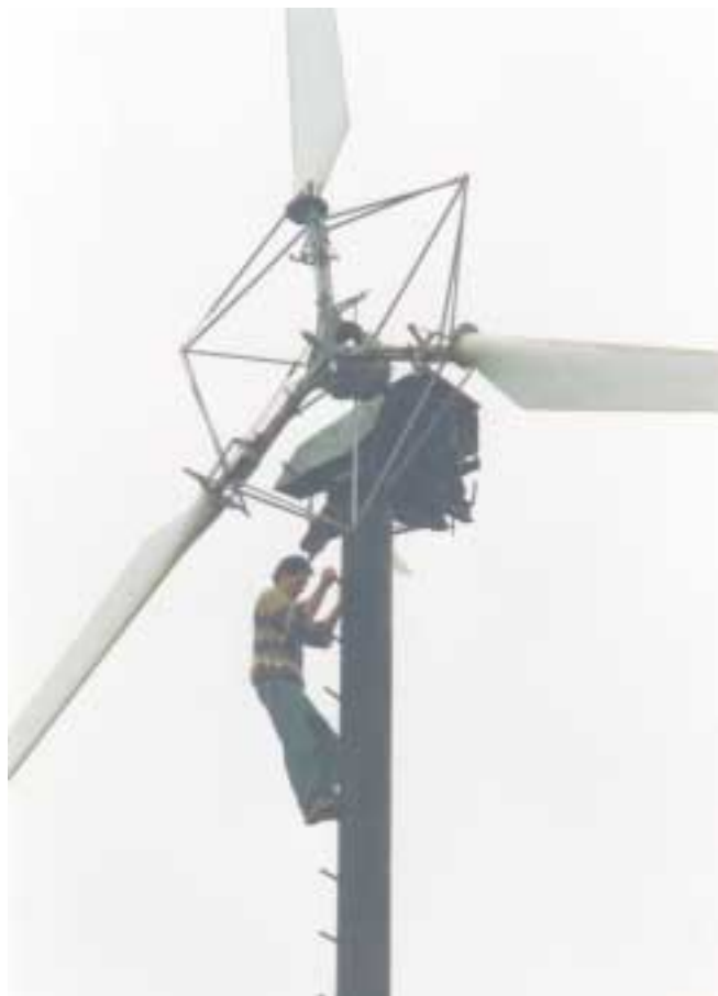
This complex wind machine built by an enthusiast in Ireland has pitch control, a gearbox, and a load-controlled synchronous alternator.
