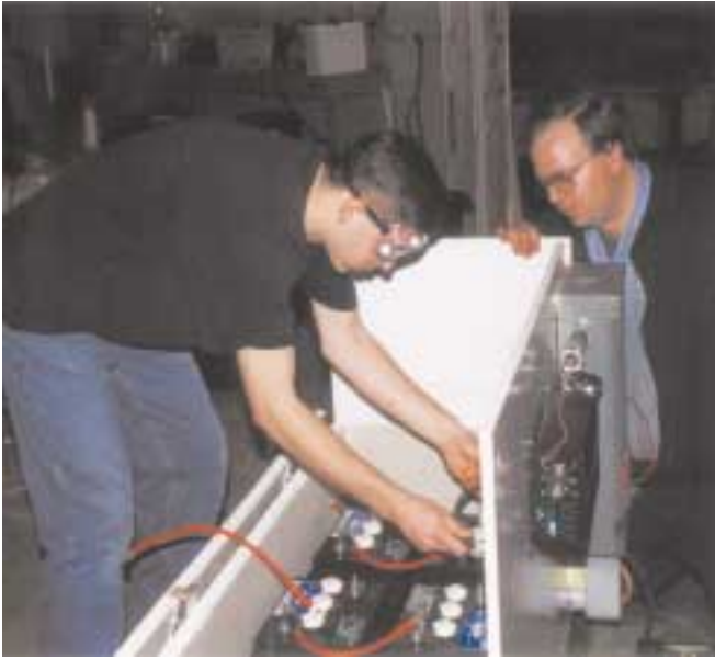
Vance works under the watchful eye of Robert from The Battery Center in Dubuque, Iowa.
