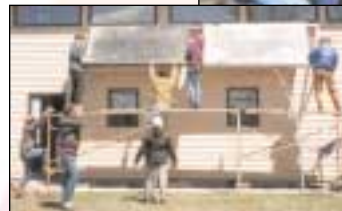
Solar Hot Water
